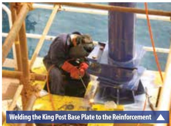
Welding the King Post Base Plate to the Reinforcement ▲
